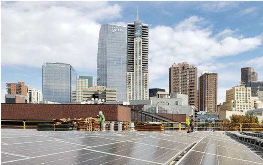
Installation of Auraria Library Solar Array
