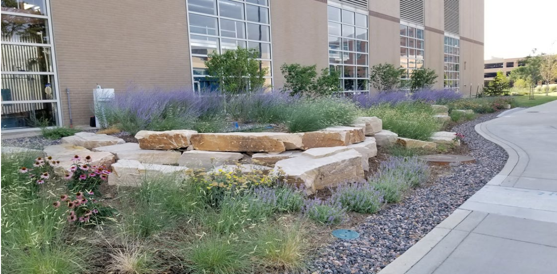
Xeriscaping Outside of Central Utility Plant
