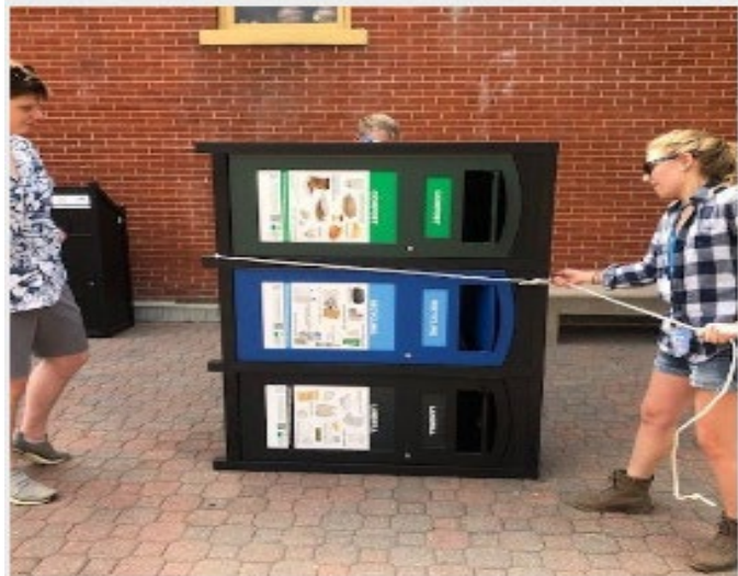
Installing Student-funded Waste Diversion Stations
